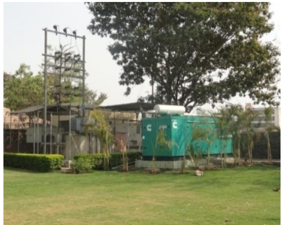
Photo no.16 272 KV Backup facility of UPS
